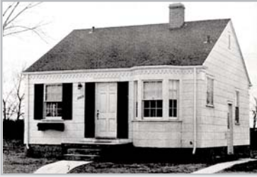
"Building Canada – Small Homes – 1946" Victory Home www.internationalmetropolis.com/
